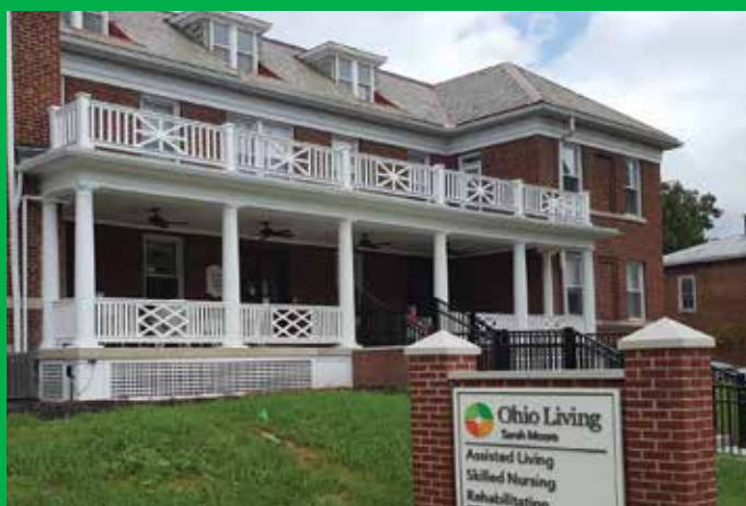
Because of a generous donation from Ohio Living Sarah Moore resident Margaret Jones, the 96 year old building was renovated with a new porch this summer.
