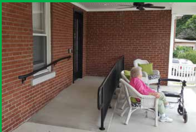
A new entrance was added with a ramp where steps used to be, making it easier for residents to access the front porch.
